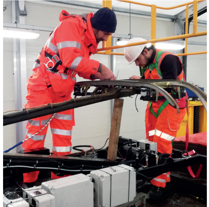
Pantograph instrumentation process for Great Western overhead line inspection (City and Brecknell Willis)
